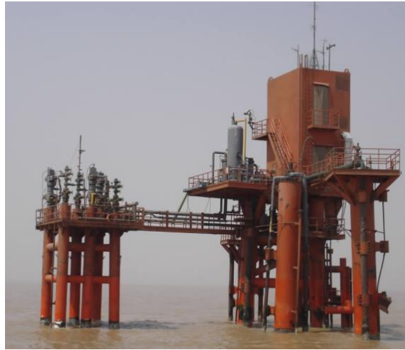
Fig. 1. Bohai Bay Jacket Platform
