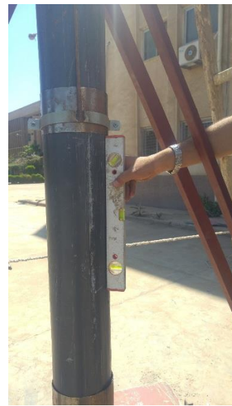
(c) Adjusting verticality
