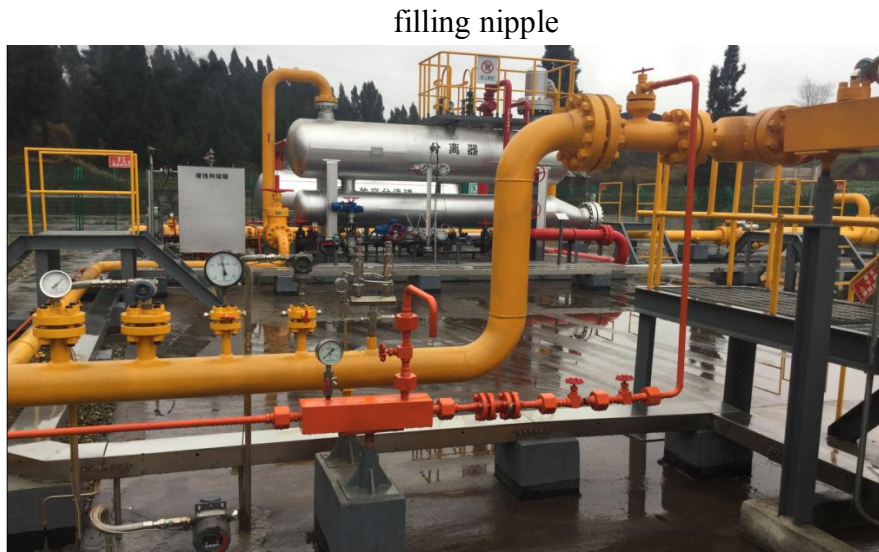
Figure 1 The position of the filling nipple
