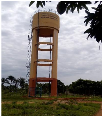
Photo 2: Hydraulic structure at Zounzonmè (Avogbanna)
