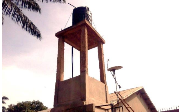
Photo 6: Water tank installed by individuals in their concession for water supply Shooting: Tchaou, april 2021
