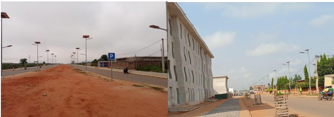
Plank4: Streetlights on site lanes Shooting , Djagoro , November 2022
