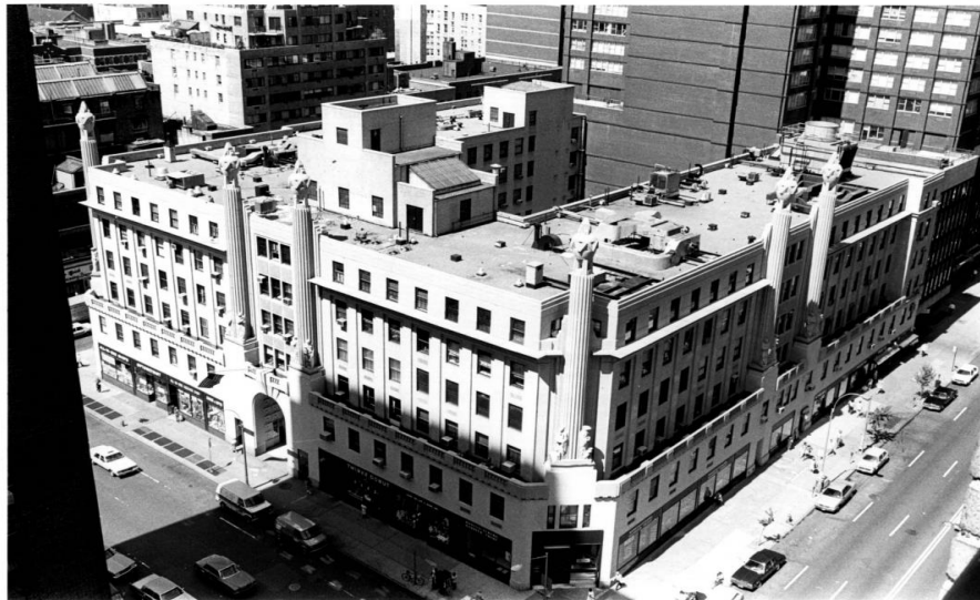
Figure 2: Hearst Magazine building, Built 1927-1925 Source: Landmarks Preservation Commission (1988)
